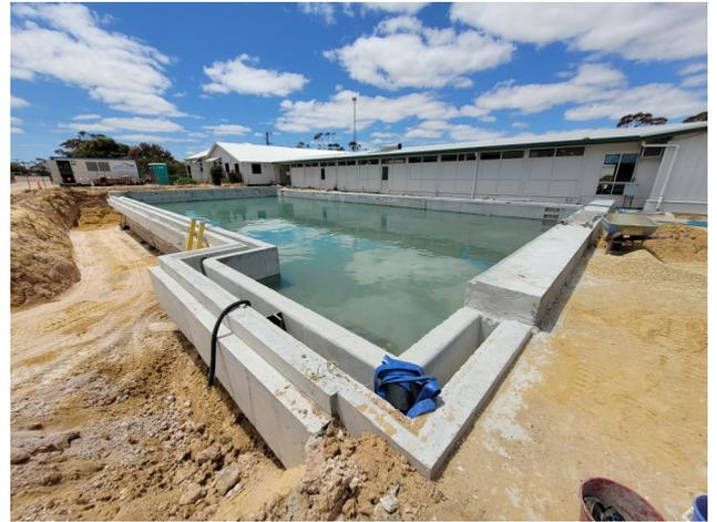
Above: Removal of the existing pool and construction of the new swimming pool facilities
