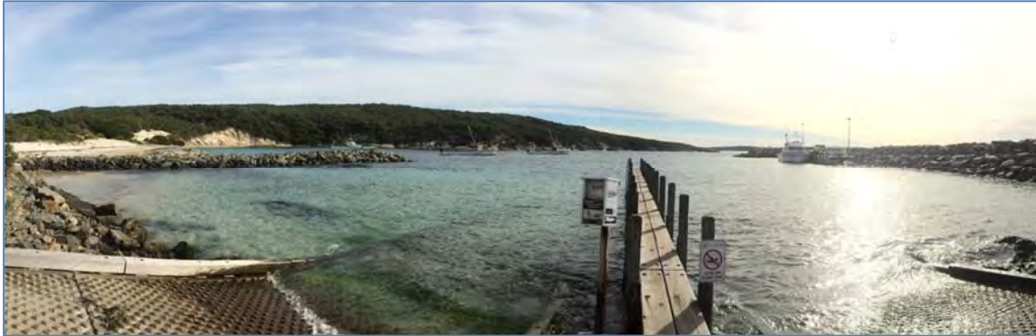
Installation of the new rock groyne (left; May 2017) is hoped to reduce sand deposits on the boat ramp area. Note erosion in rear left.
