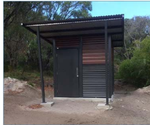
The Shire of Jerramungup has installed a new pit toilet in the camping area.
