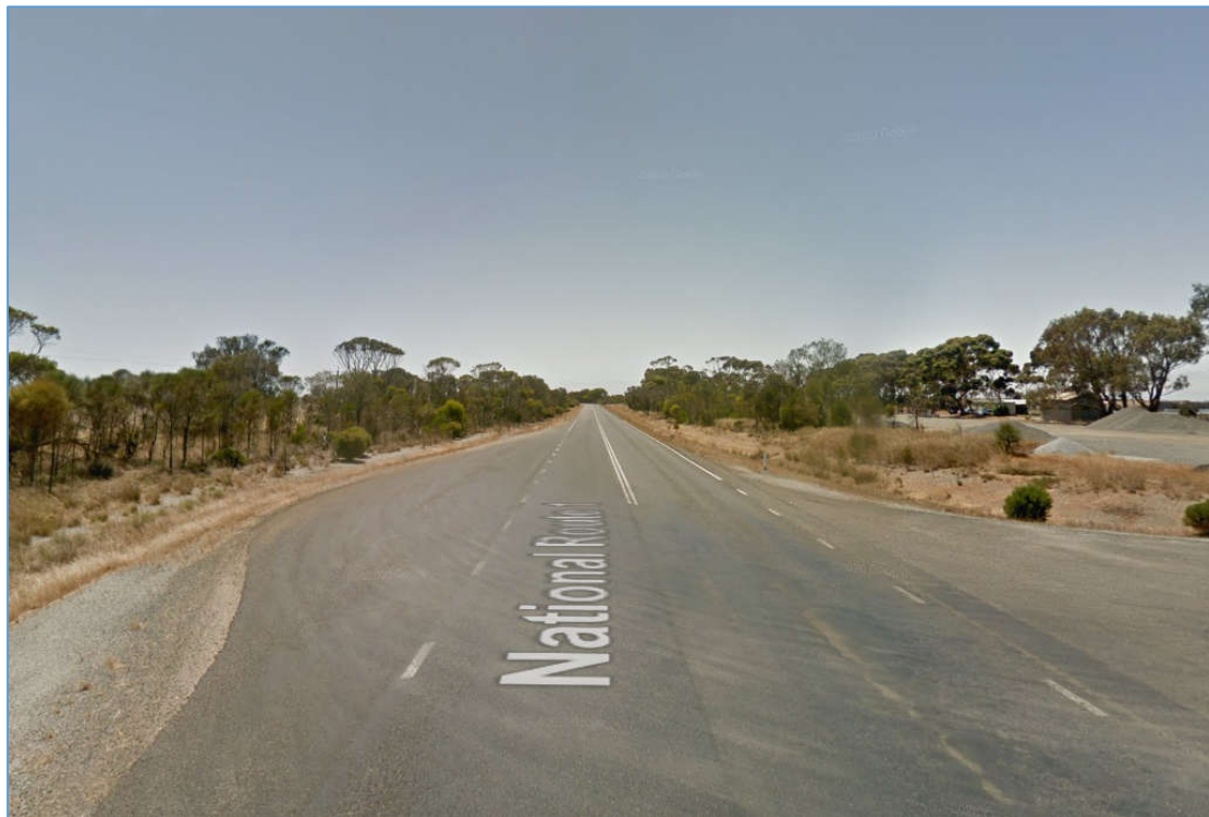
Figure 12: South Coast Hwy / CBH Exit Looking East
