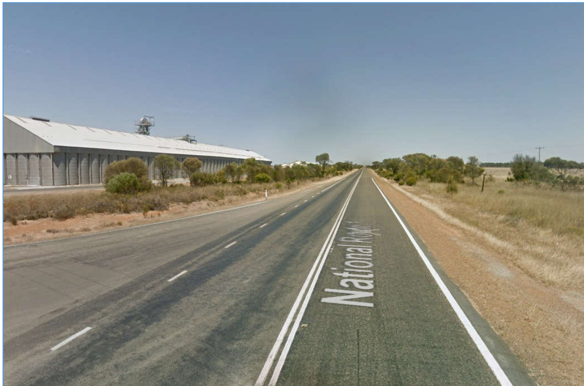
Figure 11: South Coast Hwy / CBH Exit Looking West
