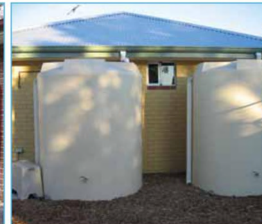
Poly domestic rainwater tanks
