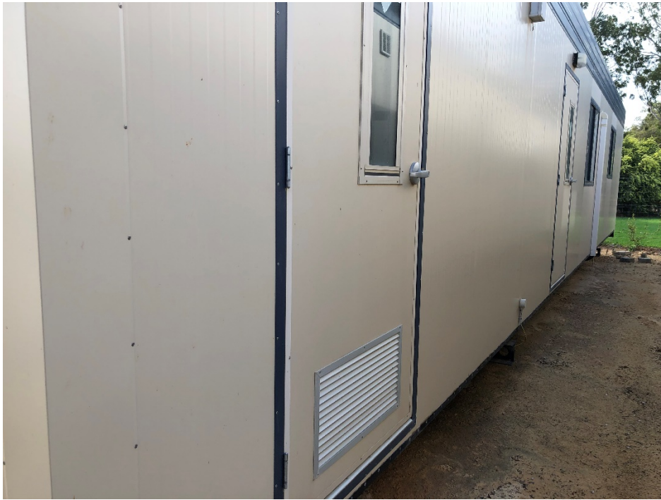
KDLU Prefabricated Building (Current Condition): Exterior
