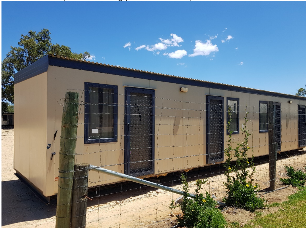
SPQ Transportable Building (Current Condition): Front elevation
