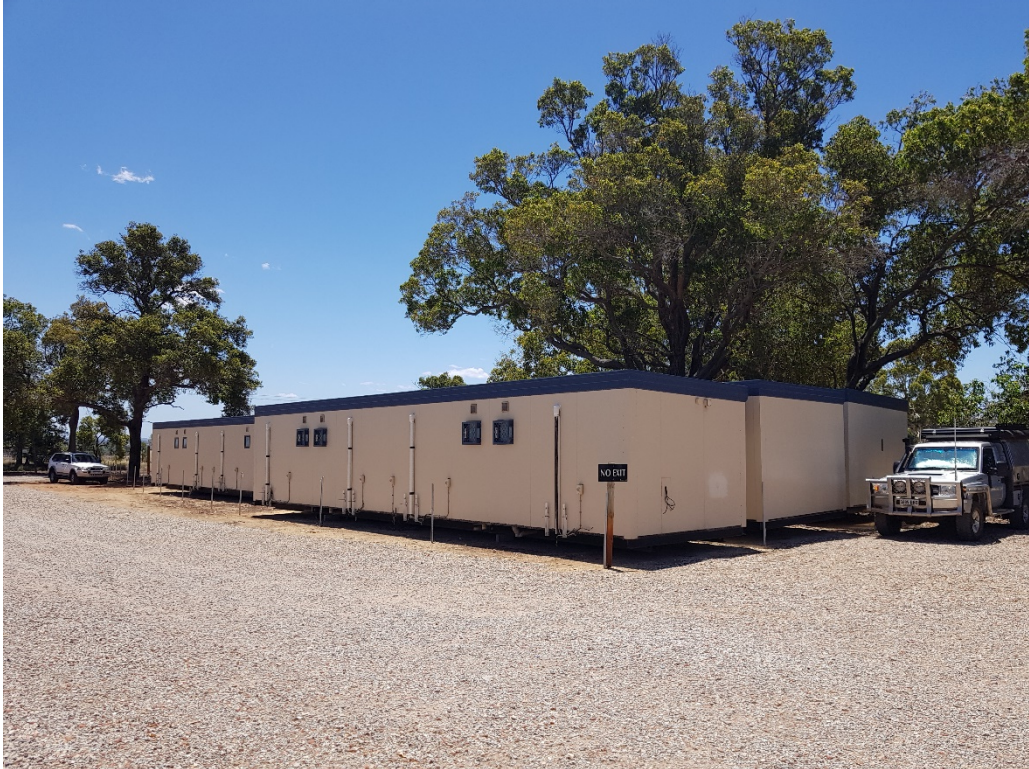
SPQ Transportable Building (Current Condition): Overall & Rear Elevation
