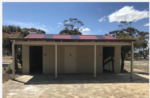
Refurbished ablution block at the Lion's Park Jerramungup
