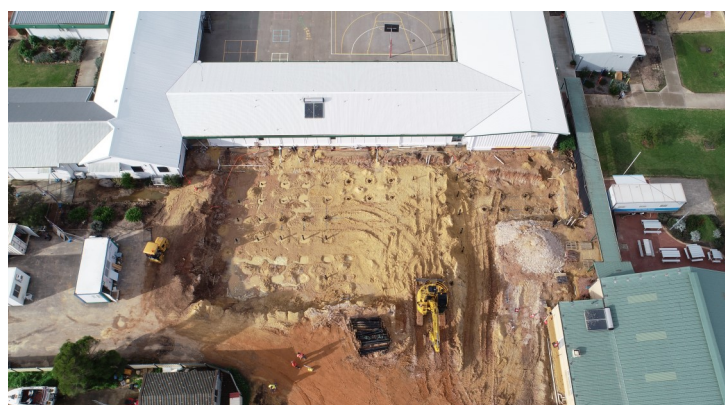
Above: Works in progress at the Jerramungup Swimming Pool Redevelopment
